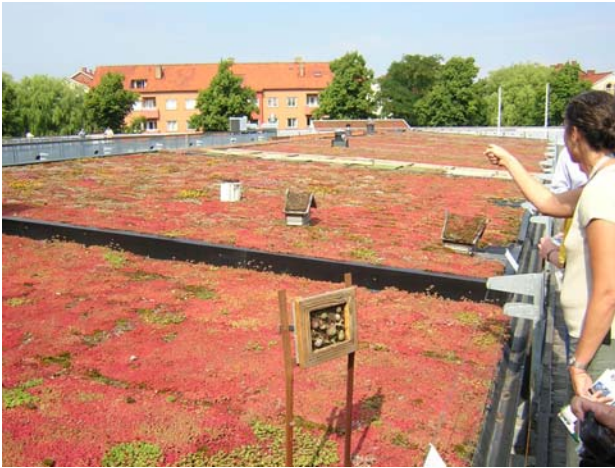
The Augustenborg botanical roof garden research centre in Malmö (Sweden) - a short drive from Copenhagen (nb. I think we should be careful not to use the term “green roofs” from now on!)
