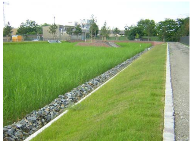
Fig.3: Stormwater treatment system, Adlershof
